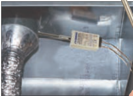
Measuring air flow and providing relay output in a ventilation hood.
